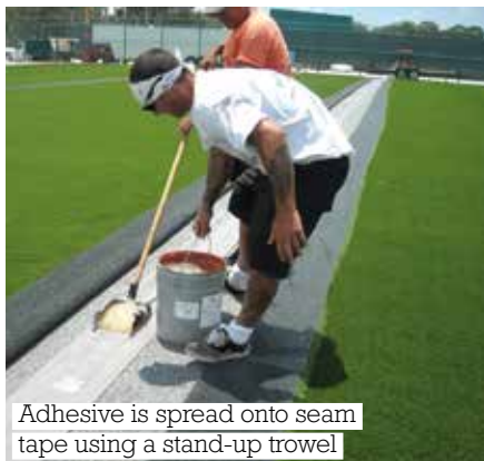
Application for cold weather turf using a stand-up squeegee
