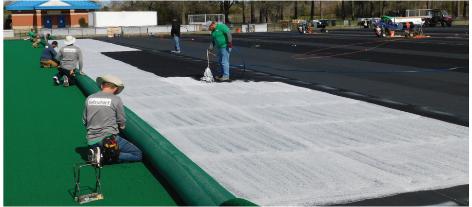
>> ADHESIVE being applied for a total gluedown with airless spray.
