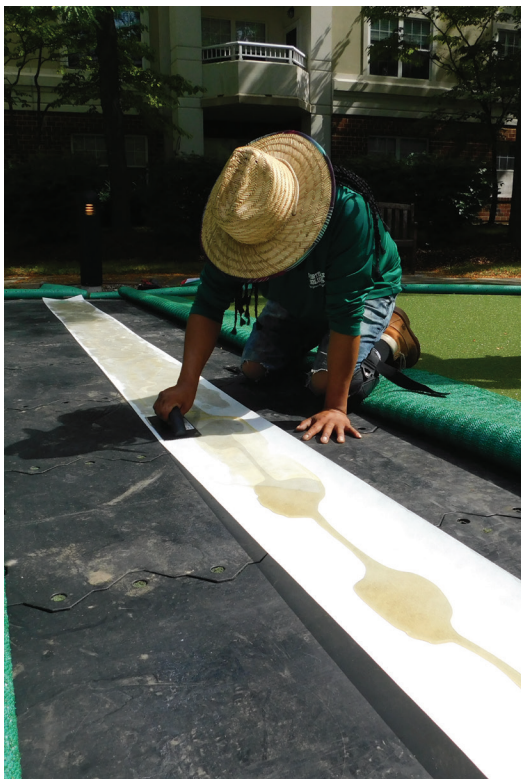
» ADHESIVE being applied to seaming tape with a kneel-down trowel.
