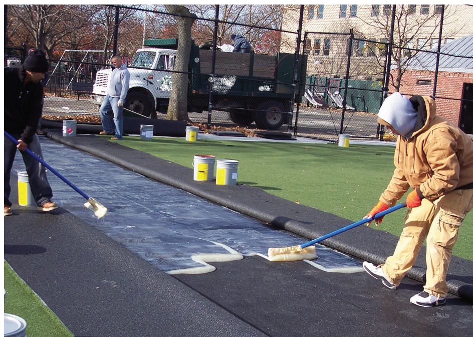
» ADHESIVE being applied to e-layer with a stand-up trowel.
