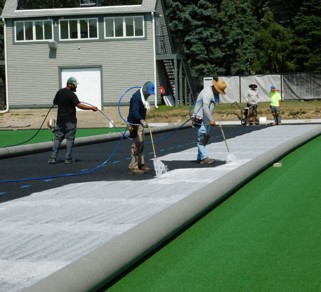
>> ADHESIVE being applied for a total gluedown by spraying.
