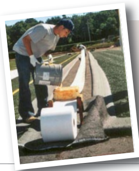
>> ADHESIVE being applied to a white seaming tap from a glue box.
