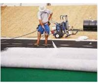
The type of spray rig that is frequently used to install these types of fields. Note that the 55-gal. drum is mounted on a portable carriage, along with the airless spray unit, so that the adhesive can be moved as the job progresses without any great effort. It also shows the adhesive being applied.
