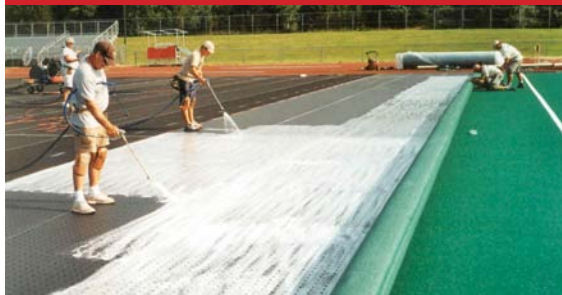
Total glue-down by spraying
